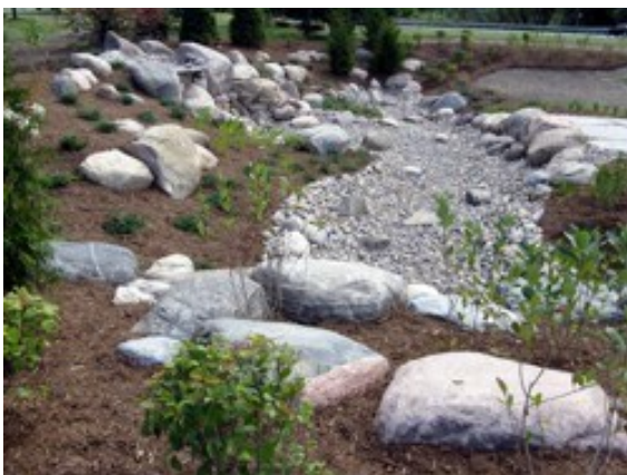
York University - Dry Swale
